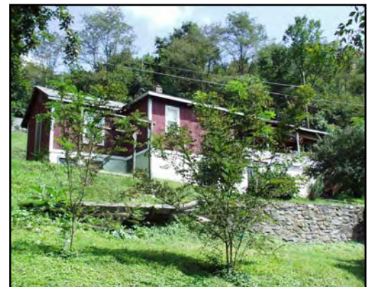
Glen Lyn project residence prior to rehabilitation.
