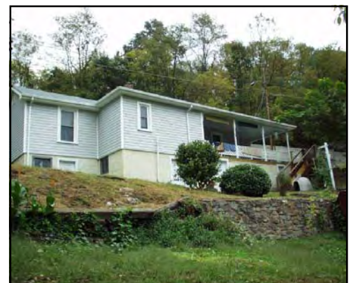
The same house after rehabilitation work.
